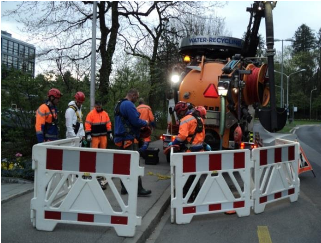
Figure 1 Cordoned-off & identified work area
