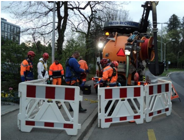
Figure 2 Cordoned-off & identified work area
