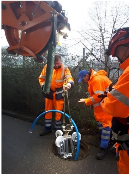
Figure 4 P360 being lowered into manhole
