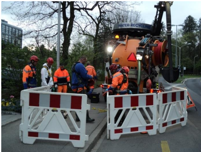
Figure 3 Cordoned-off & identified work area
