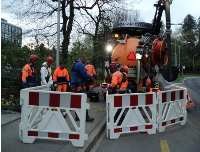
Figure 1 Cordoned-off & identified work area
